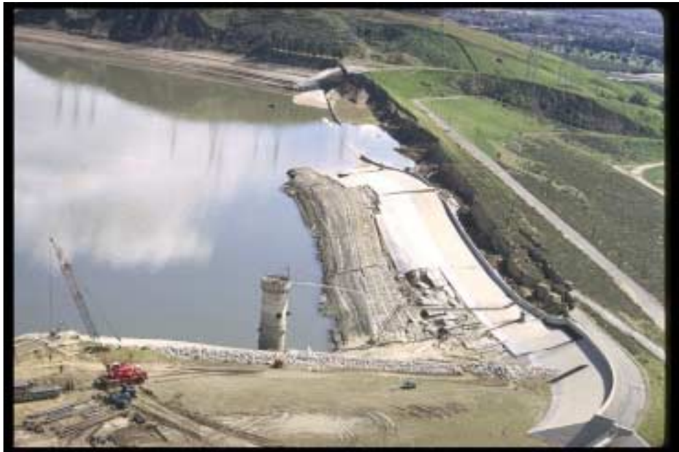
The upstream face and crest of the Lower San Fernando Dam slid into the Lower Van Norman Reservoir in 1971, prompting the evacuation of 75,000-80,000 residents downstream.
