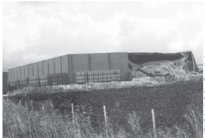
Figure 41 - Pallets of canned goods stored in this building fell off the shelves during the 1989 Loma Prieta earthquake and pushed out the concrete wall of this Hollister warehouse.
