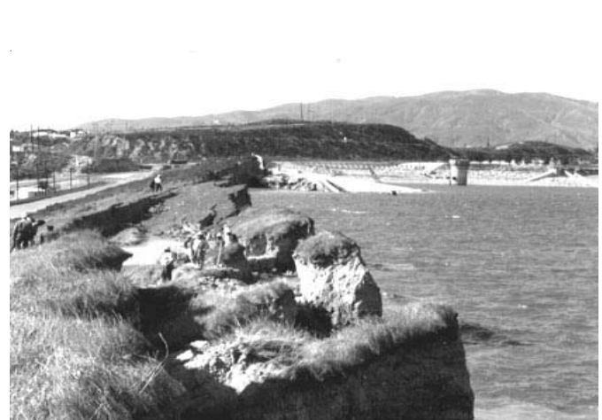
Figure 69 - Lower San Fernando Dam that was badly damaged by the 1971 San Fernando Earthquake.
