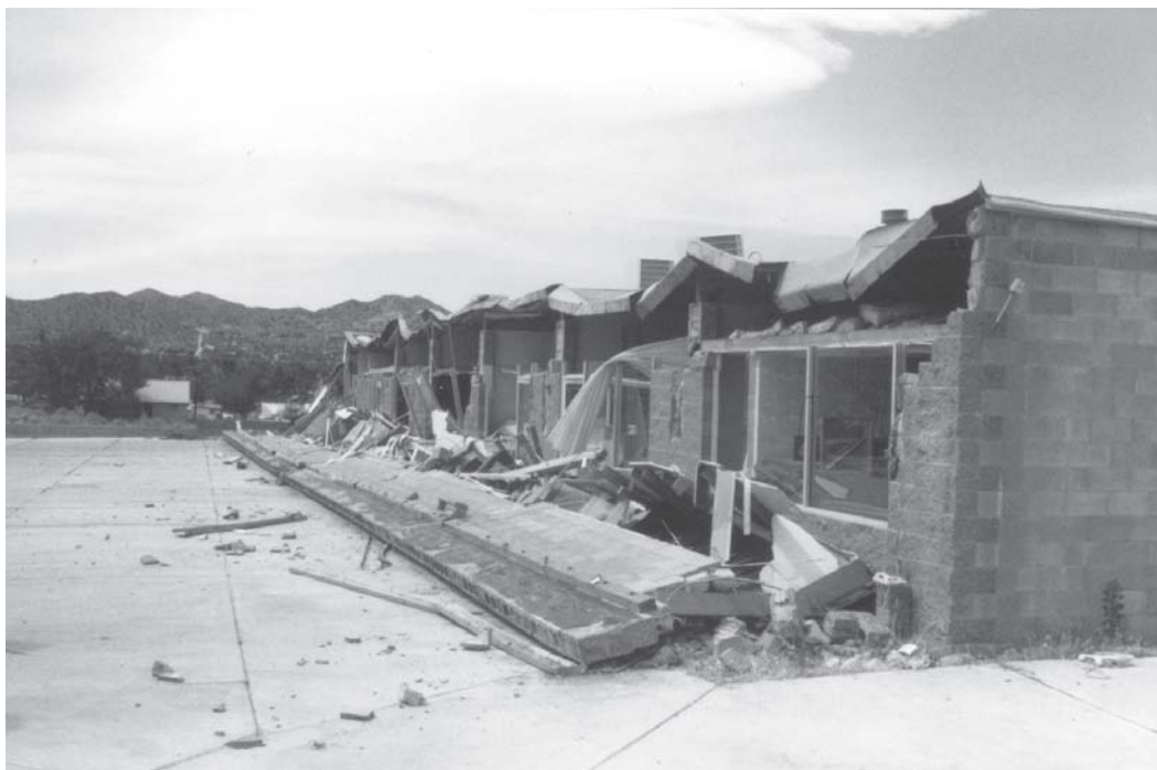
Figure 15 — Wall Anchors Can Prevent Failures Like This. Even newer buildings are not immune to earthquakes. This reinforced masonry strip mall was built in the 1980's but did not comply with the building code. The wall anchorage failed in the 1992 Landers Earthquake. Its front wall fell into the parking lot.
