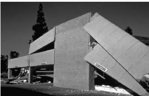
Figure 5 - Concrete Parking Structure Collapse.
