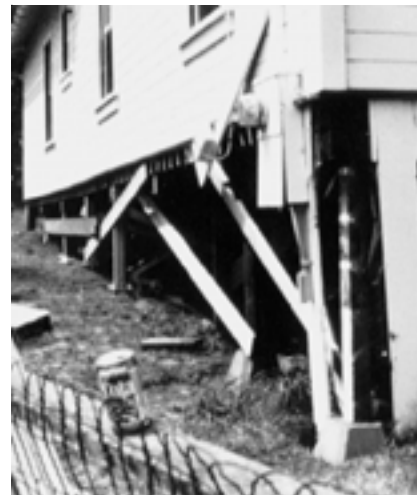
Figure 18 - The pier-and-post foundation under this home shifted during a recent earthquake.
