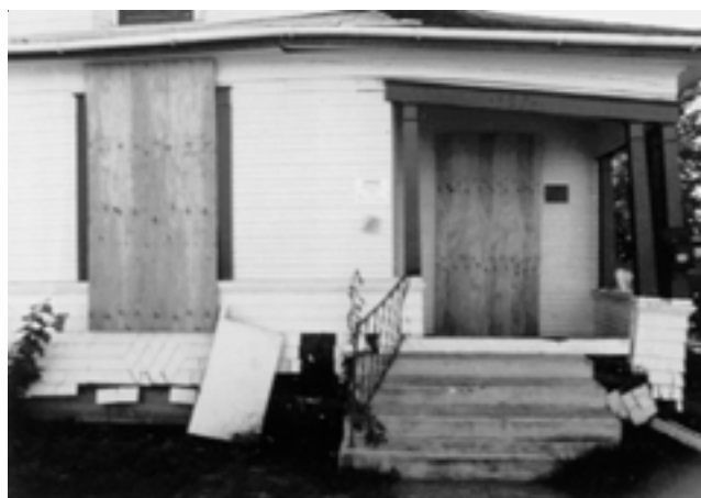
Figure 13 - This home wasn't bolted and slid off its foundation. Sometimes the damage can be so bad that houses have to be demolished.
